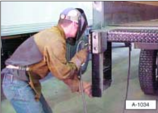
Illustration 20b. Tack weld dock bumpers.
